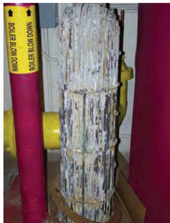
After 90 Days Untreated Water
